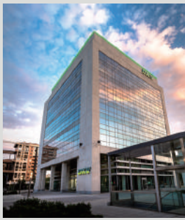
HQ Mansion of DKV, Spain
